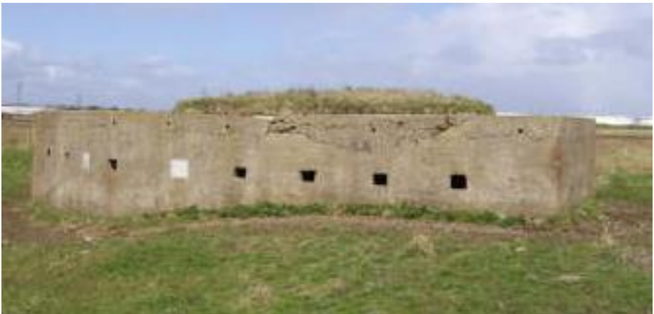
Section posts were essentially hardened trench works. Constructed to bullet-proof standard, they were long and had a large number of embrasures. Shelves of wood or concrete were fitted below the embrasures in the principle direction.
