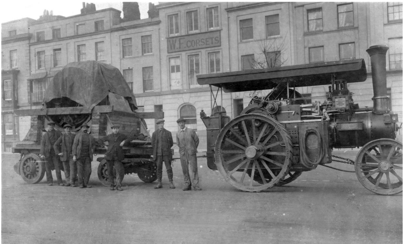
Alternator en route to Portsmouth Power Station
