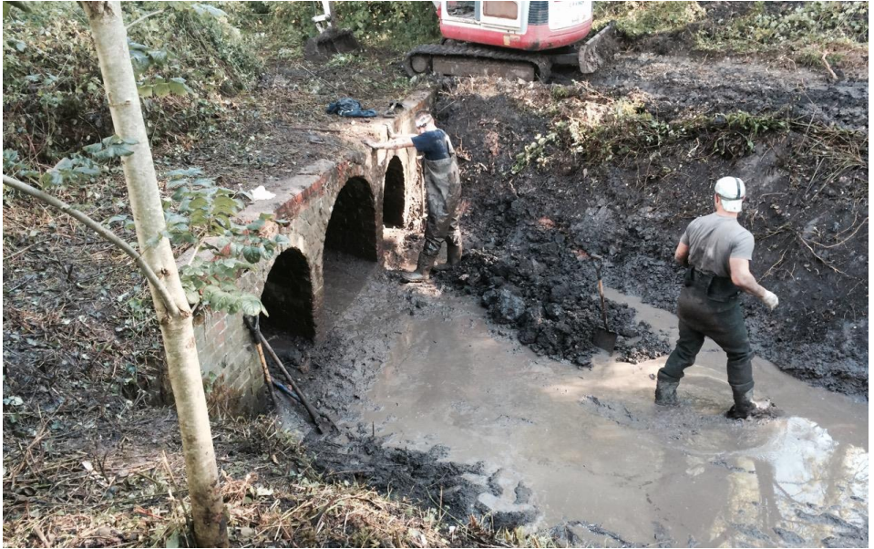
Rowlands Castle Sling culvert clearance in September 2015
