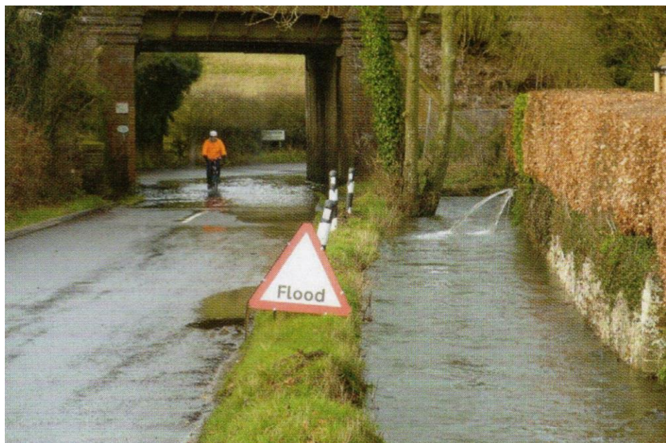
Dean Lane End. The ditch and overflow from the fields towards Finchdean on the other side of the arch. The water being pumped the houses (possibly an old well) to the right.
