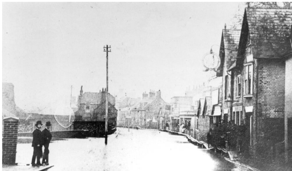
North Street flooded in the 1880s. Originally the Lavant Stream flowed down North Street and Elm Lane in the open with bridges across. Note the raised walkway which appears to be a permanent feature.
