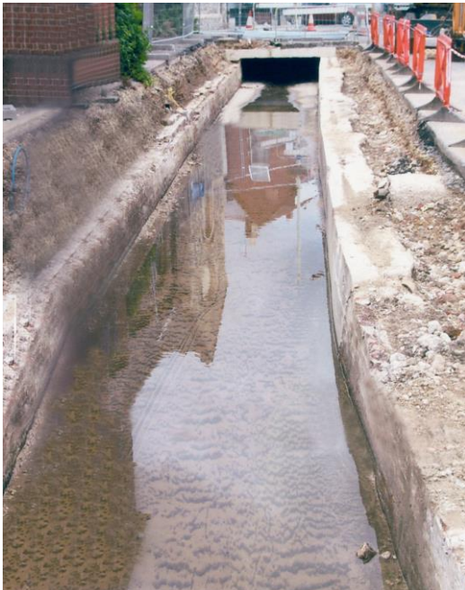
The Lavant Stream exposed in Elm Lane during the replacement of the roof of the culvert. Early 2000s.
