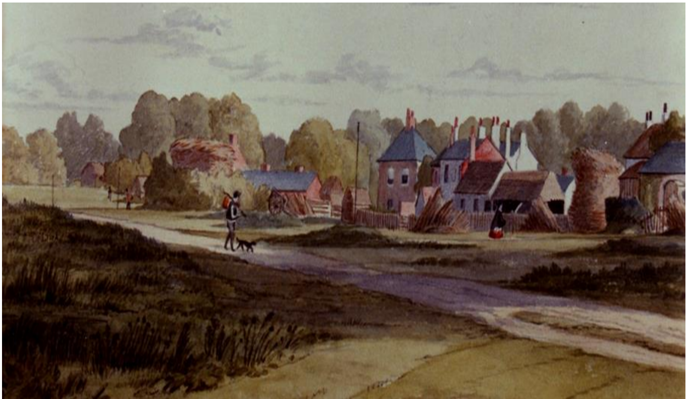
Durrants from behind the Staunton Arms. In the little gardens where fruit trees and bushes are mingled with kitchen herbs, a heap of brushwood is piled upon the common to indicate that the winter fuel was provided.
