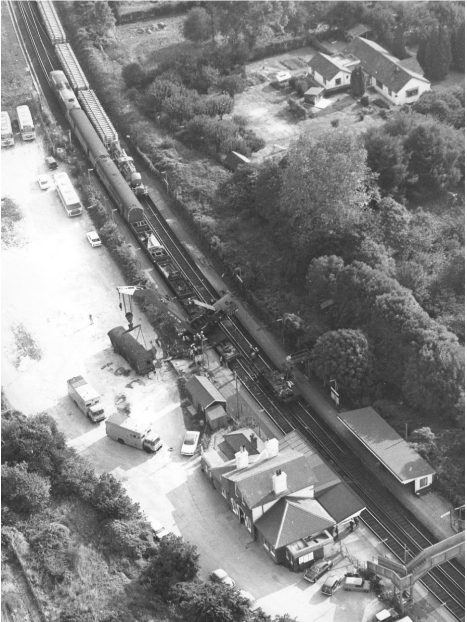
Aerial view showing the scene at the station: the wrecked brake van, the damaged mess van, the toppled crane and wagons loaded with pre-assembled new track that ran away.
