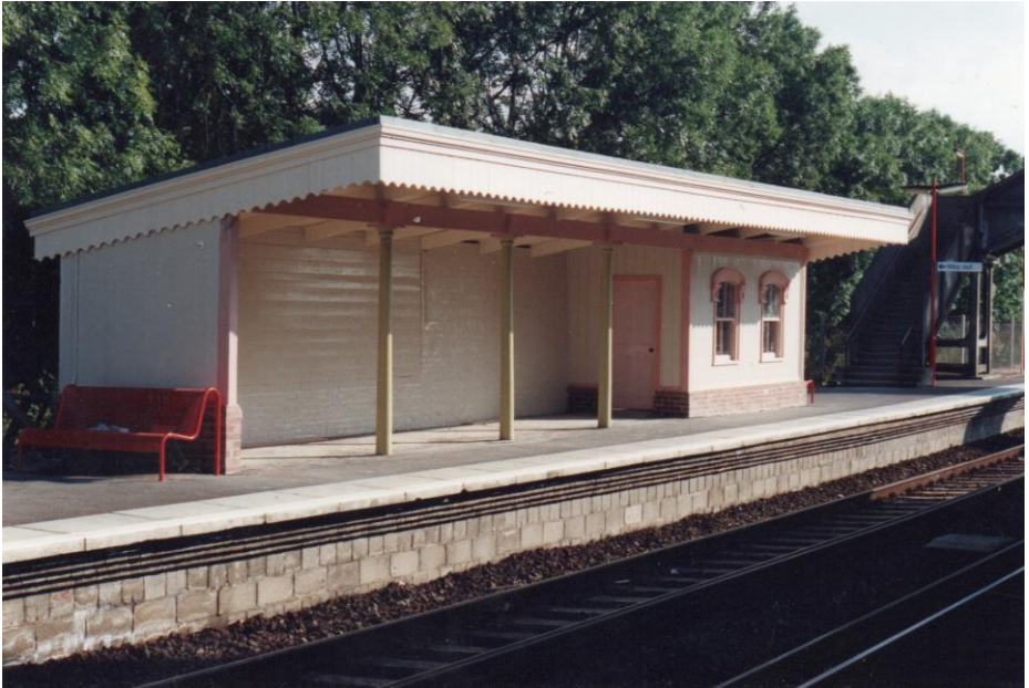
14 April 1992. The new shelter on the Down side. Paul Marshman
