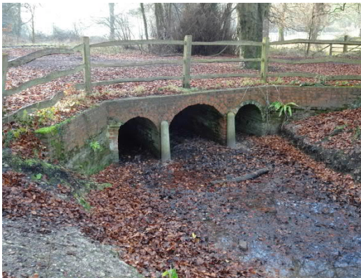
Entrance to the 42 metre long culvert
