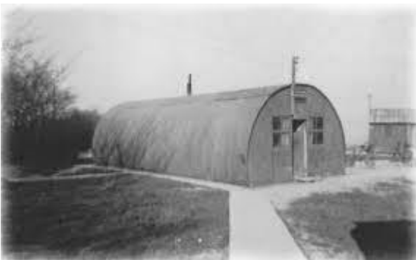
Erected Nissen Hut
