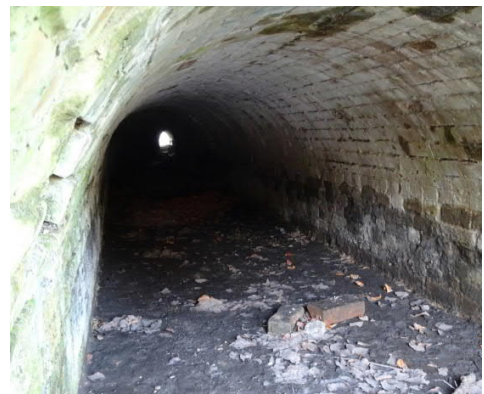
Inside the culvert after clearance
