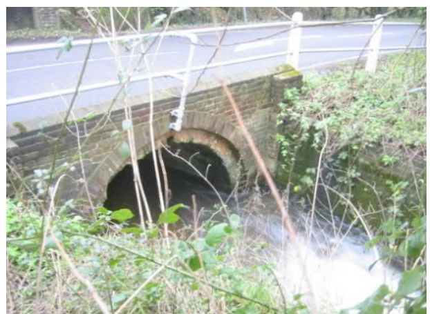
The Culvert under Emsworth Common Road
