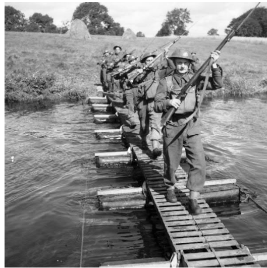
Men of the 8th Sherwood Foresters cross a river using a small kapok pontoon bridge, Dunadry in Northern Ireland, 28 August 1941.
