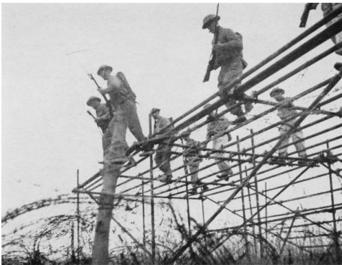
Scaffolding stage may have looked like this
